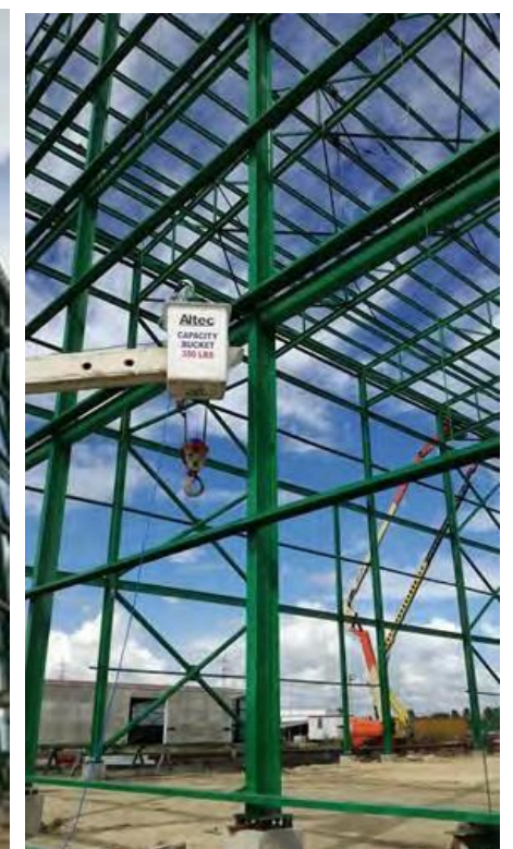
INSTALLATION OF STRUCTURAL BUILDING FOR COAL STORAGE IN SAN PEDRO BIOENERGY PLANT 45.8M X 40 M X 23.40 M
