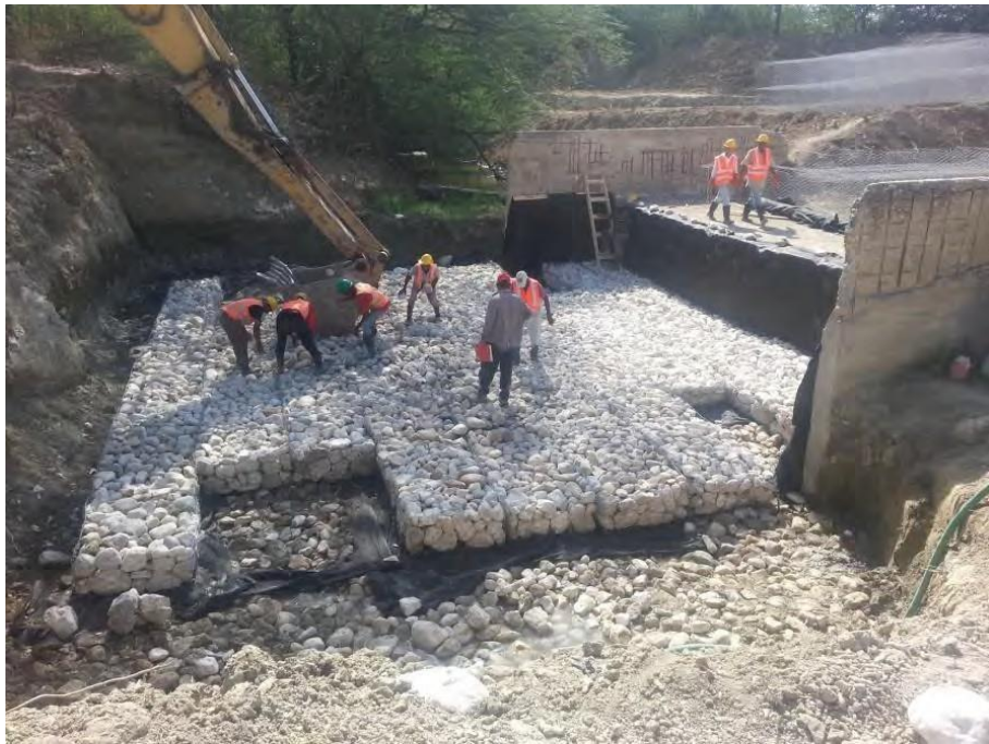
CONSTRUCTION OF WALLS AND PLATFORMS OF GAVIONS AND EROSION CONTROL, CANAL CRISTÓBAL, PROJECT LOTE 1
