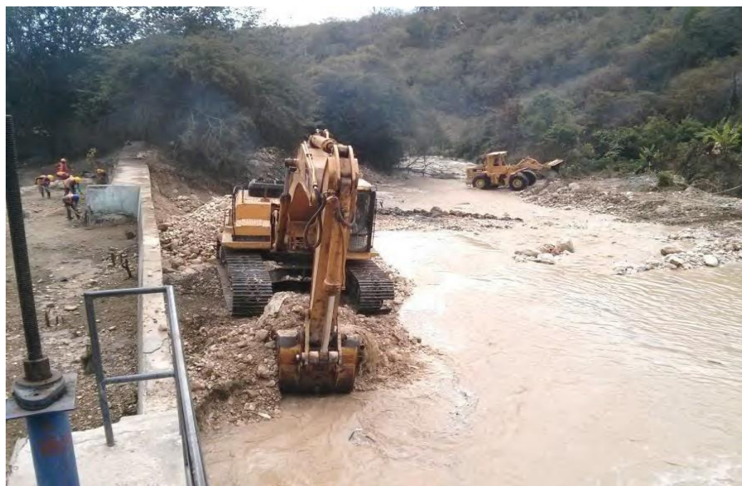
WORK WITH HIGH FREATIC LEVEL CAMBRONAL WATERWAY - LOT 1
