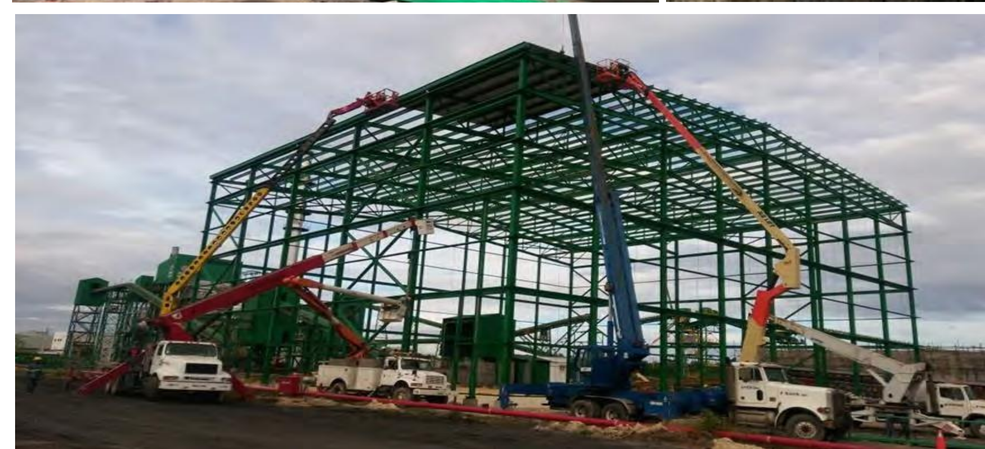
INSTALLATION OF STRUCTURAL BUILDING FOR COAL STORAGE IN SAN PEDRO BIOENERGY PLANT 45.8M X 40 M X 23.40 M
