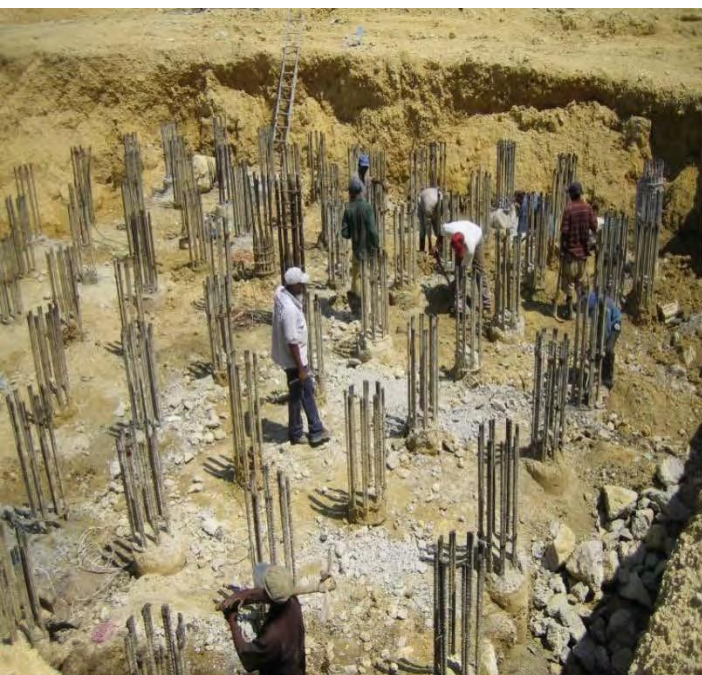
DRILLING AND EMPTYING "IN SITU" OF 915 PILOTS OF REINFORCED CONCRETE, PROJECT LINE NO. 1, METRO DE SANTO DOMINGO
