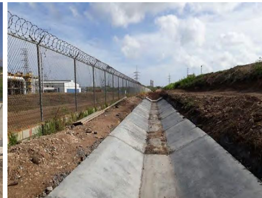
CONSTRUCTION OF DRAINAGE IN QUISQUEYA I AND II PLANT
