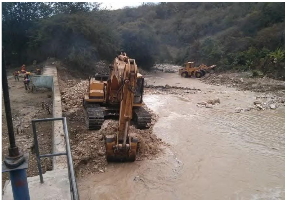
ELIMINATION OF BODY MATERIALS OF THE RIVER WATER UP OF THE DAM, LEVELING OF THE RIVER IN THE REMOVAL AREA, WATER UP AND WATER DOWN THE DAM, CAMBRONAL CHANNEL - LOT PROJECT 1
