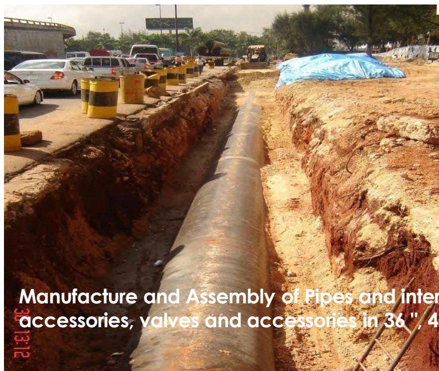
Installation of carbon steel pipe system, butterfly valves and expansion joints, drains
