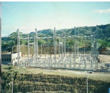
Bulla-Monción Substation of 138kv - 50 MVA
