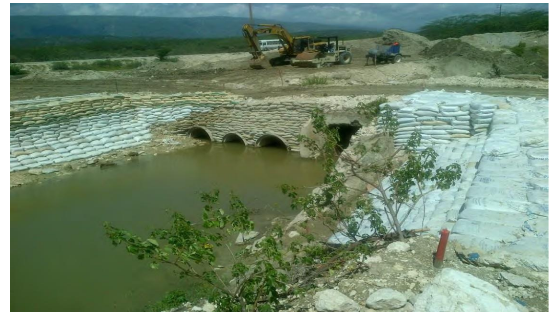
WORKS OF WALLS OF CONTAINMENT IN SUCKS STABILIZED IN CEMENT, STRUCTURE IN MATTRESS OF GAVIONES FOR CHANNEL CHRISTOBAL, PROJECT LOT 1.
