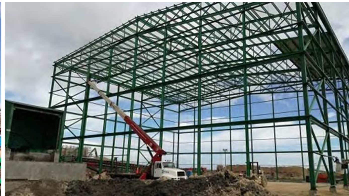
INSTALLATION OF STRUCTURAL BUILDING FOR COAL STORAGE IN SAN PEDRO BIOENERGY PLANT 45.8M X 40 M X 23.40 M
