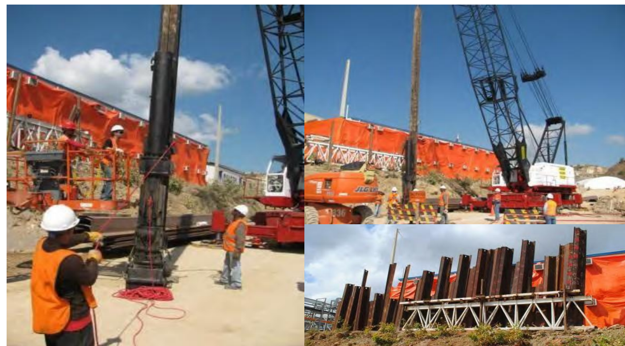
CIVIL WORKS AND INSTALLATION STEEL SHEETS (SHEET PILING), PROJECT F336, BARRICK GOLD PROJECT.
