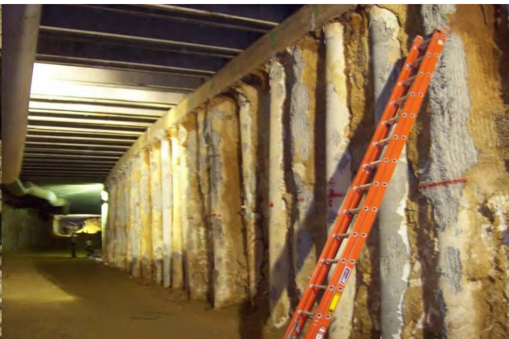
DRILLING AND EMPTYING "IN SITU" OF 915 PILOTS OF REINFORCED CONCRETE, PROJECT LINE NO. 1, METRO DE SANTO DOMINGO
